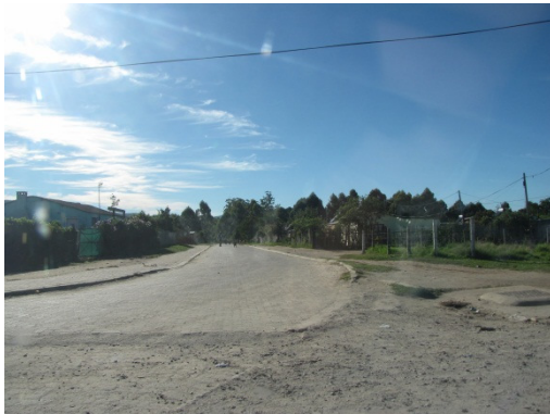
Road condition along Walker Road
