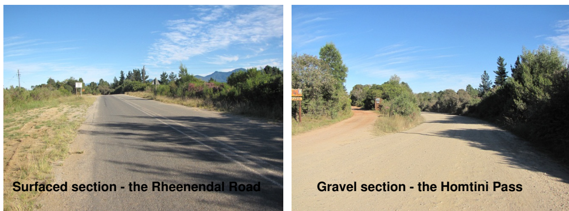
Figure 3: Current condition of the MR355
