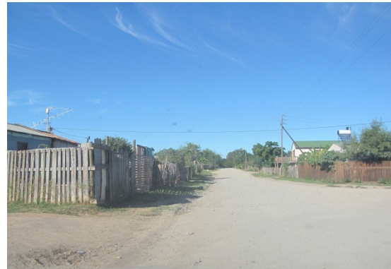
Gravel section along Walker Road
