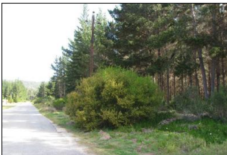
FIGURE 7: EXISTING MINOR ROAD 6913 ALONG EASTERN BOUNDARY OF PORTION 18
