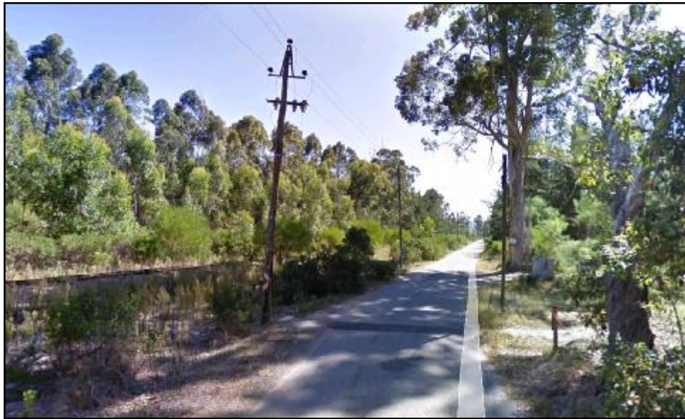
FIGURE 8: MINOR ROAD 6912 AND RAILWAY LINE ALONG THE SOUTHERN BOUNDARY OF THE APPLICATION AREA
