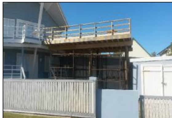
FIGURE 16: PATIO BEING CONSTRUCTED ABOVE GARAGE ON ERF 75
