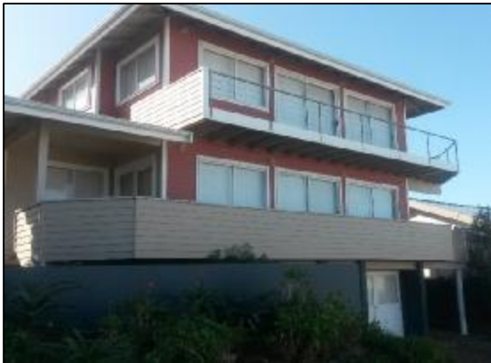
FIGURE 3: STRUCTURE ON ERF 141
