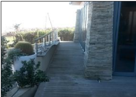
FIGURE 9: DECK SOUTH OF COVERED VERANDA
