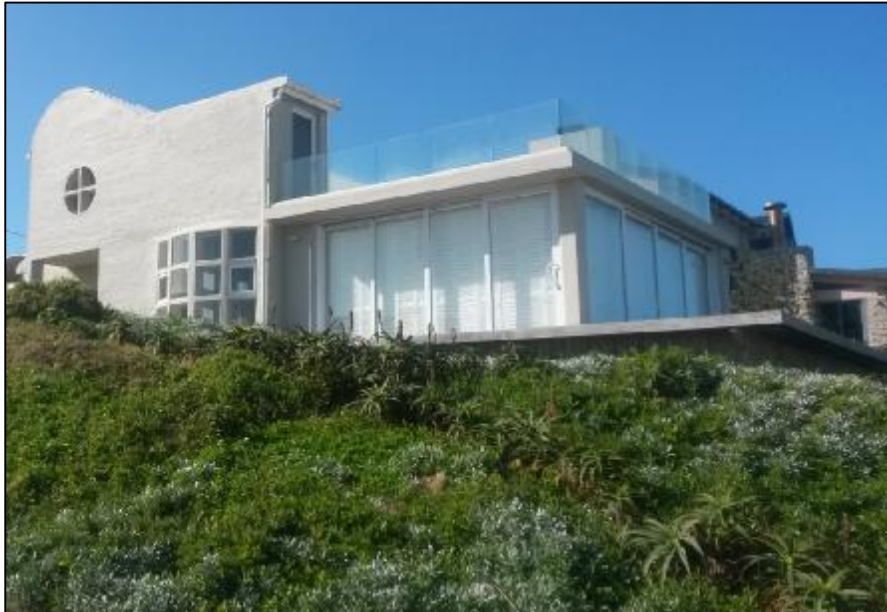
FIGURE 14: DECK ON NEIGHBOURING ERF 74
