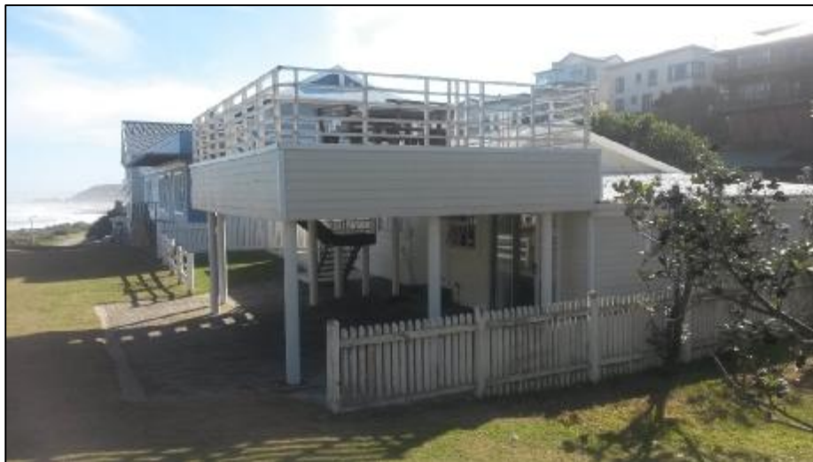
FIGURE 6: DECK AREA LOCATED ABOVE CAR PORT AREA ON ERF 148
