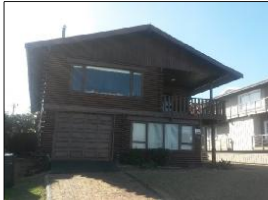
FIGURE 4: ERF 80 NEIGHBOURING SUBJECT PROPERTY TO EAST
