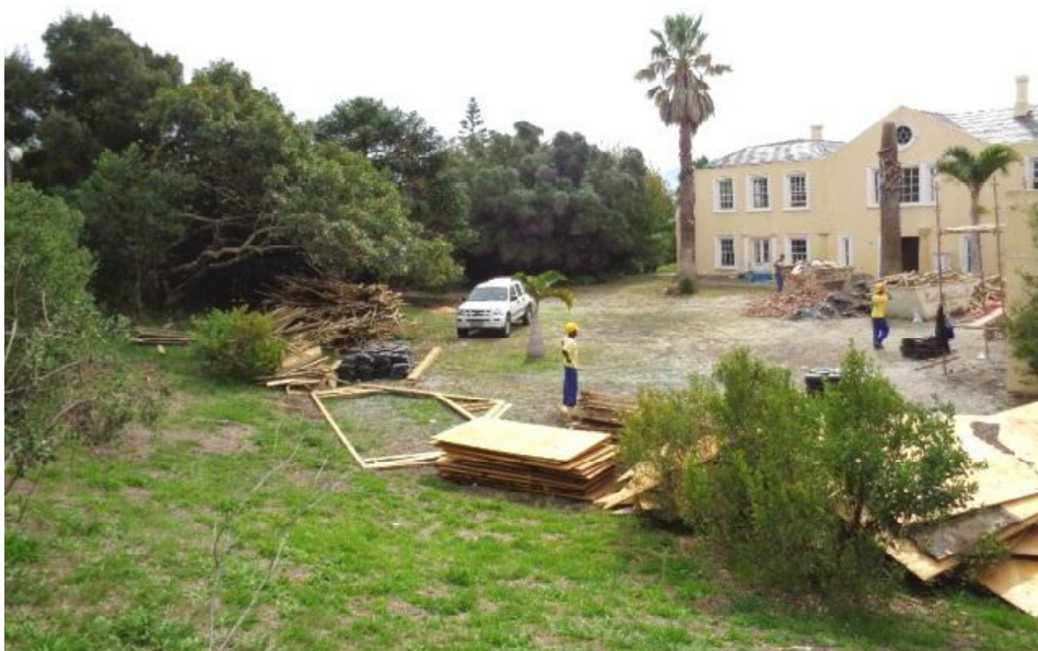
Photo 2 Wooded area behind the manor house (under renovation).
