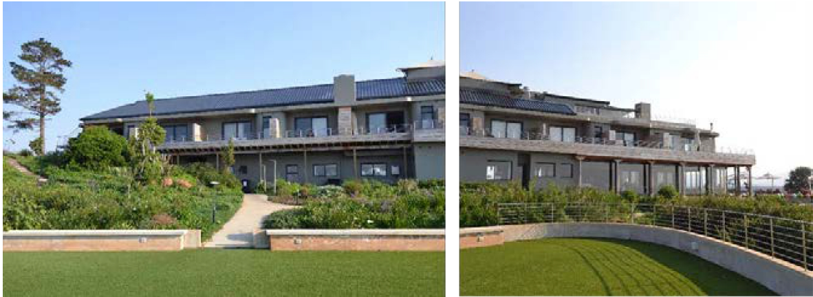
Figure 13: Views of the Manor House post alteration (Continued...)
