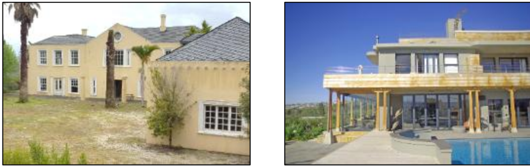
FIGURE 10: THE MANOR HOUSE – THEN AND NOW
