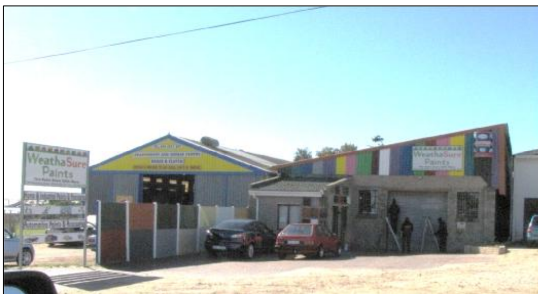
FIGURE 22: WEATHA SURE PAINTS AND ROADWORTHY CENTRE ON SCHOEMAN STREET
