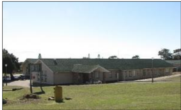
FIGURE 19: MOSSEL BAY HOSPITAL ON ERF 3215
