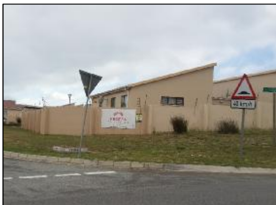
FIGURE 20: GROUP HOUSING ON ERF 12272
