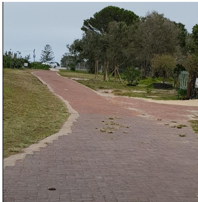
FIGURE 4: INTERNAL ROAD TOWARDS THE EXIT
