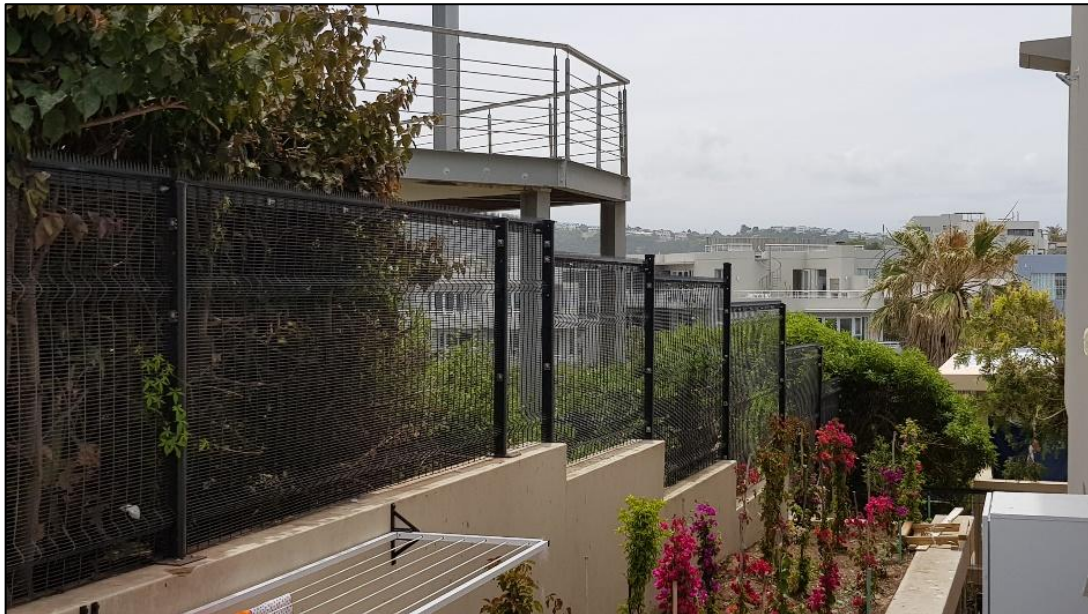
FIGURE 28: BOUNDARY WALL TO THE WEST OF THE APPLICATION AREA
