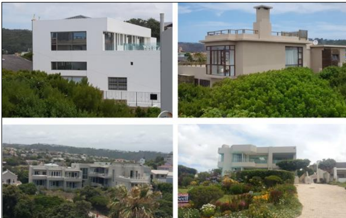
FIGURE 13: LARGE, FLAT ROOFED STRUCTURES IN CLOSE PROXIMITY TO THE APPLICATION AREA
